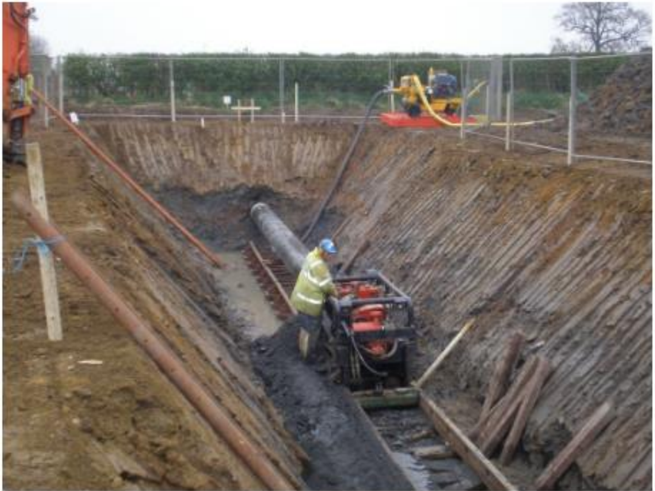
Figure 3-40: Auger Boring at a Road Crossing
