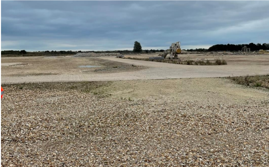
Figure 3-21: Former TGT Site and Option 1 for Theddlethorpe Facility
