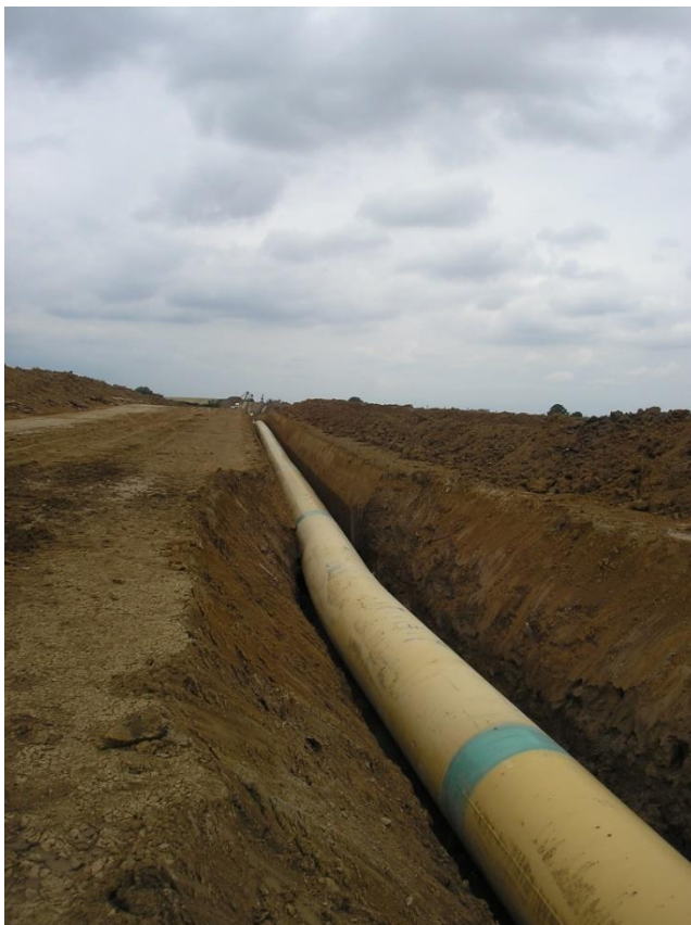
Figure 3-39: Open Cut Technique
