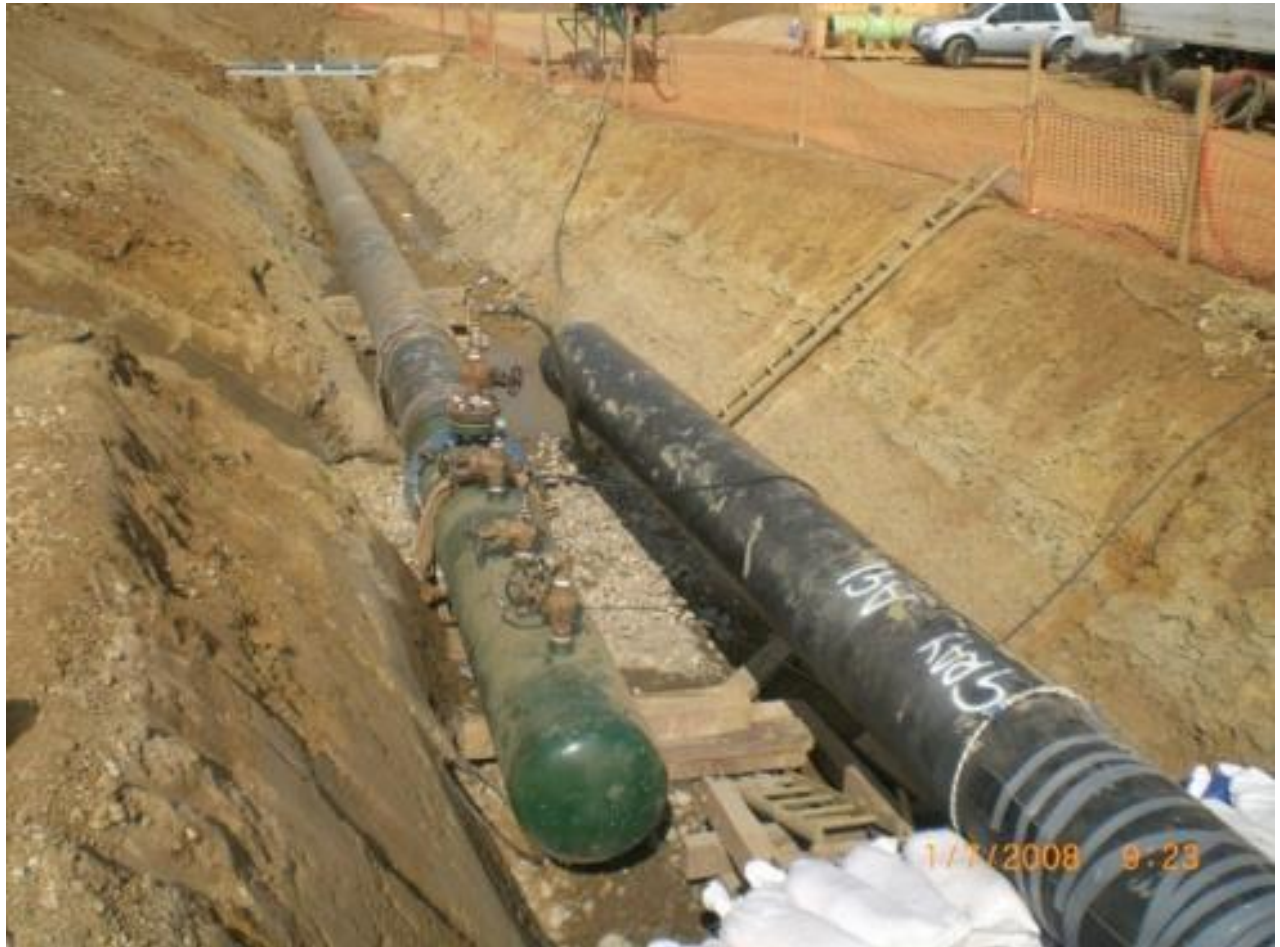
Figure 3-44: Hydrotesting in Operation
